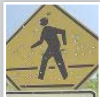
03 Special crossing treatments (warning signs, beacons, etc. (5.1)
