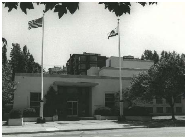
LEFT: Set within a residential area, the North Point Sewage Treatment Plant is comprised of a grouping of buildings designed a late iteration of the Streamline Moderne style. Built in 1950, the extant building features rounded overhangs, banding at the windows and roofline, and stepped back upper stories. Landscape features include a generous setback, planters, and a sidewall that mimics the fenestration configuration. Photo: 1976 Architectural Survey field form
