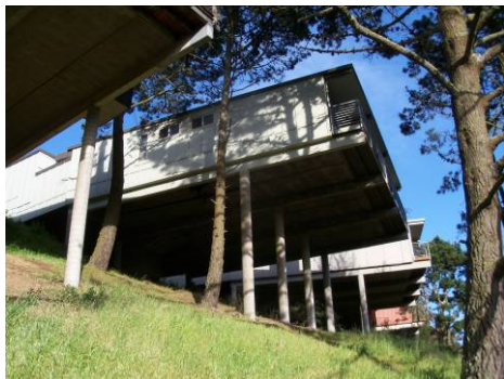
Perched on concrete pilings, a dozen Second Bay Tradition boxes jut out over the steeply sloped hills above Glen Canyon. Developed by the Galli Construction Co. and designed by architects Hayes & Smith, the single-family dwellings were constructed in 1964.
