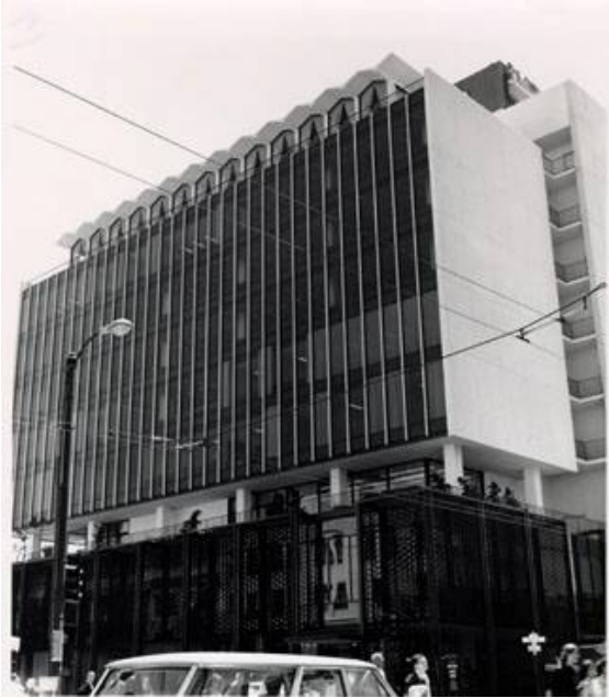
The flagship 1963 Bay View Federal Savings on Mission Street (left) features glass cladding, a barrel-vaulted roofline, a midlevel terrace, and, at the lower stories, metal sheathing. The anodized sheathing (above) mimics the shape of an eagle, the bank's corporate logo. The bank sits on squat structural supports, producing a floating effect at the ground level. It was designed by FTM Associates. Photo: San Francisco History Center, San Francisco Public Library; Mary Brown, San Francisco Planning Department
