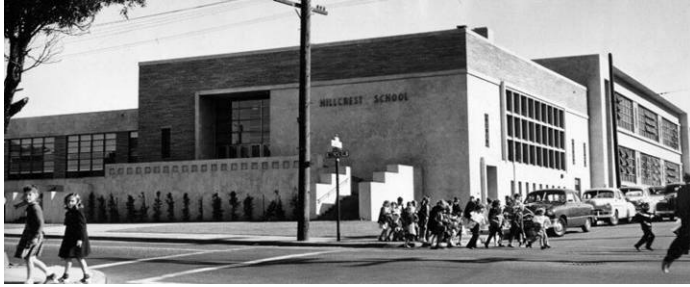
LEFT: Hillcrest Elementary School (1951) on Silver Avenue.
