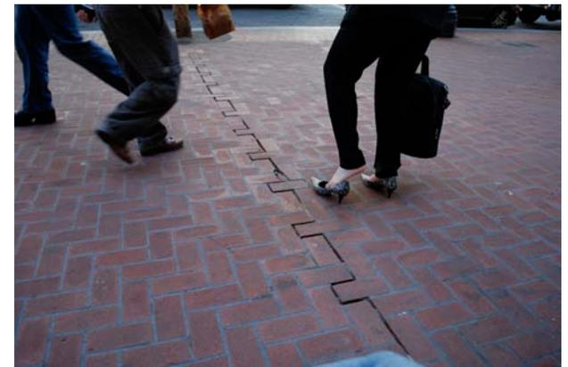
When unrepaired, the expansion joints are a hazard to high-heeled shoes.
