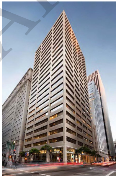
180 Montgomery Street, 1979 (CBRE.us)
