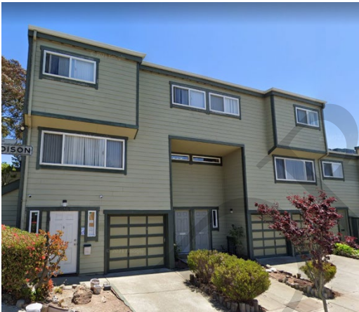
Diamond View Apartments, 296 Addison Street (Google Maps).
