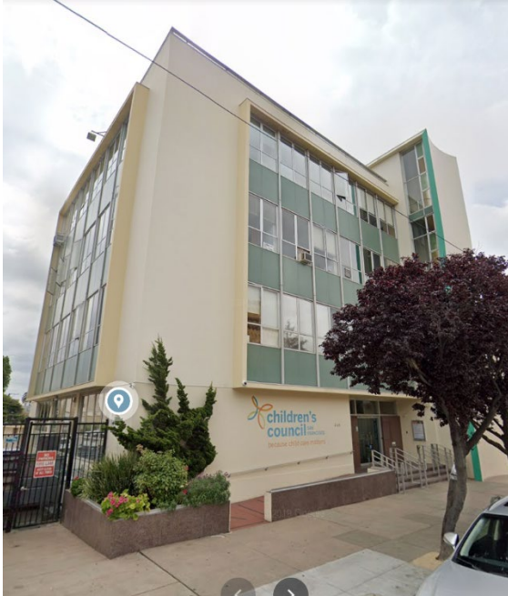
445 Church Street, 1959 (Google Maps).
