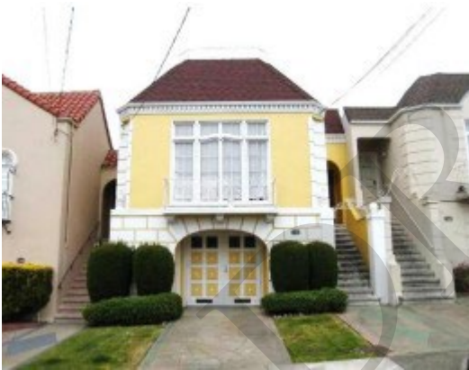
1454 32 nd Avenue, (Sunset District Residential Builders, 1925-1950 Historic Context Statement).
