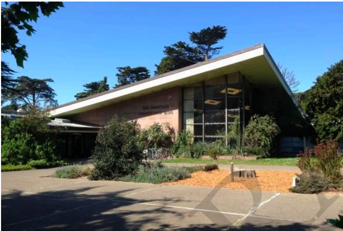
San Francisco County Fair Building (formerly Hall of Flowers), (San Francisco Recreation and Parks).
