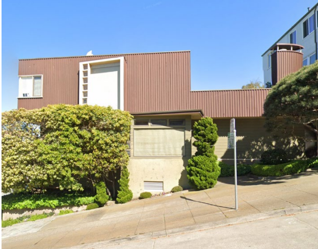
Roos House, 2660 Divisadero Street, 1938 (Google Maps).
