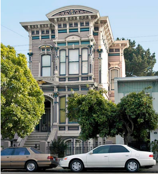
Havens Mansion and Carriage House, 1381 South Van Ness Avenue, 1884, San Francisco Landmark #125 (NoeHill).
