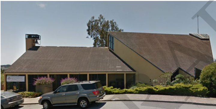
Shepard of the Hills Lutheran Church, 395 Addison Street, 1966 (Google Maps).
