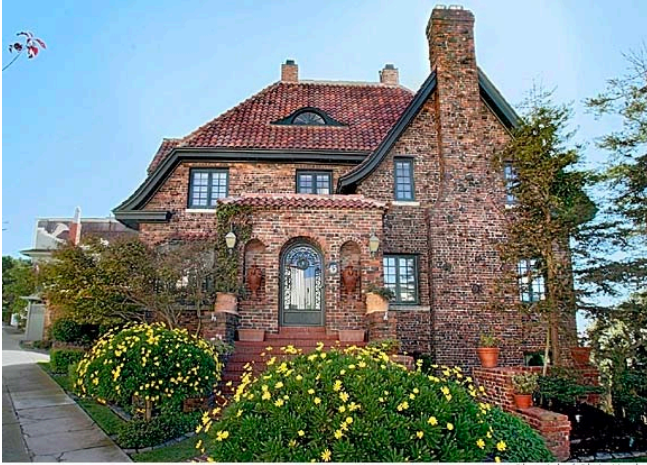
1916 Clinker Brick Residence, (Chris Hardy for San Francisco Chronicle).
