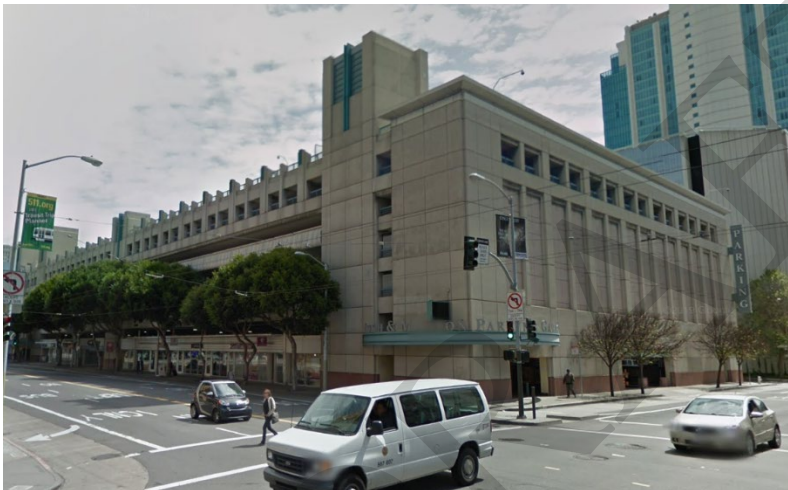
5 th and Mission Parking Garage, 899 Mission Street, 1995 (Google Maps).
