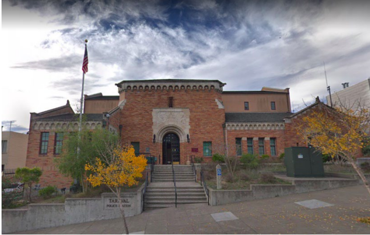
Taraval Police Station, 1930 (SFHeritage.org).
