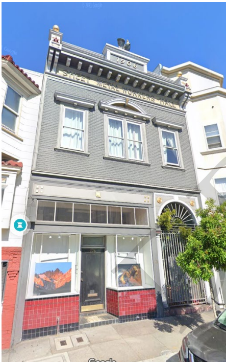
Sheet Metal Workers Hall, 224-26 Guerrero Street, 1906 (Google Maps).
