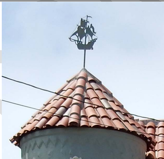
weathervane on a turret cap
