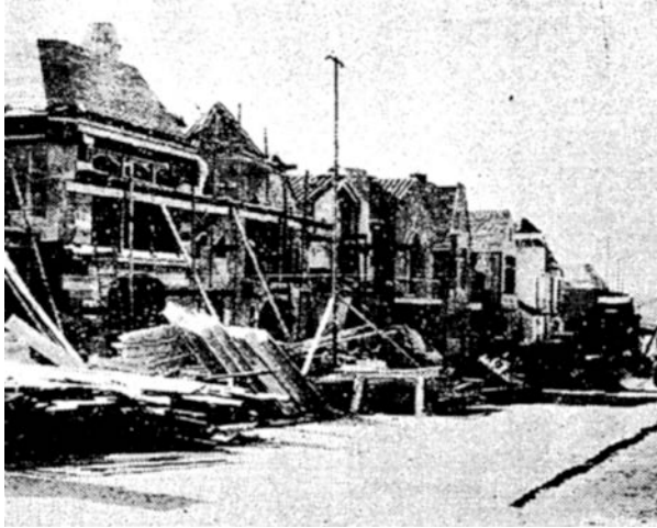
Construction along 34 th Avenue in 1933.
