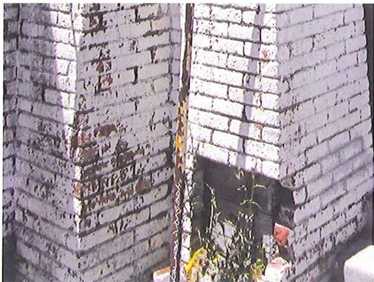
Photograph 2. Southeast Corner, Deteriorated Brick Veneer
