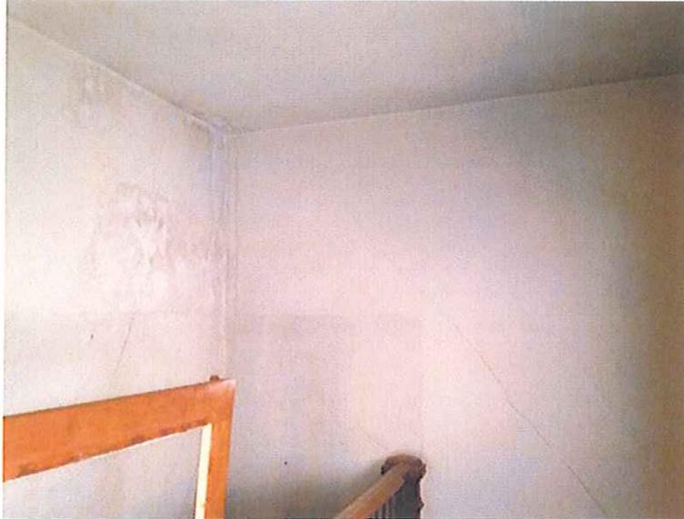
Photograph 11. Interior of Northeast Stairwell Showing Cracks
