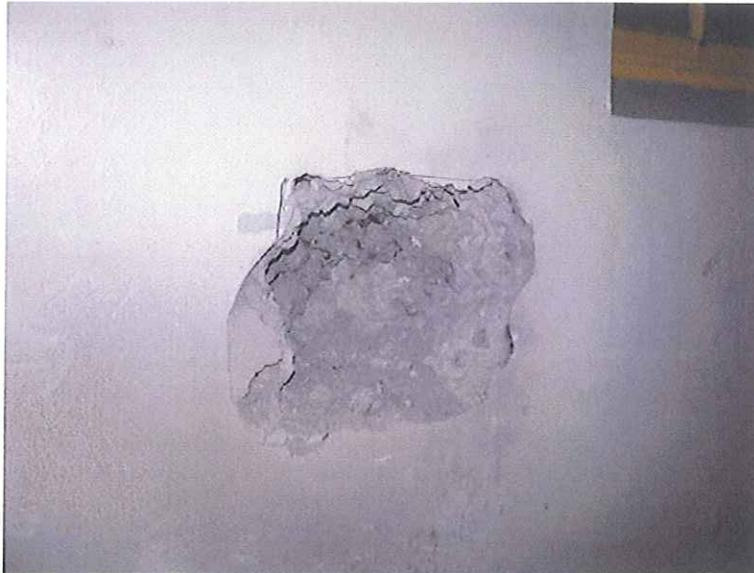
Photograph 13. Chipped South Wall in Basement Showing no Reinforcement in Concrete Wall
