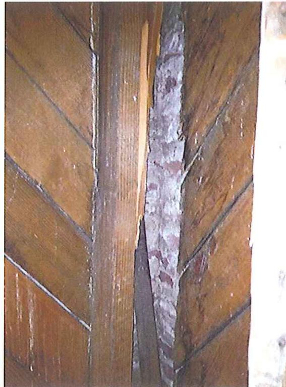
Photograph 6. South Wall Interior Showing Damaged Framing
