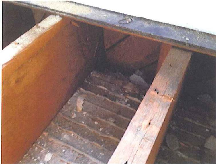
Photograph 15. Exposed Mezzanine Floor Framing and Diagonal Wall Sheathing
