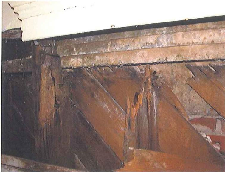
Photograph 7. South Wall Interior Showing Damaged Framing
