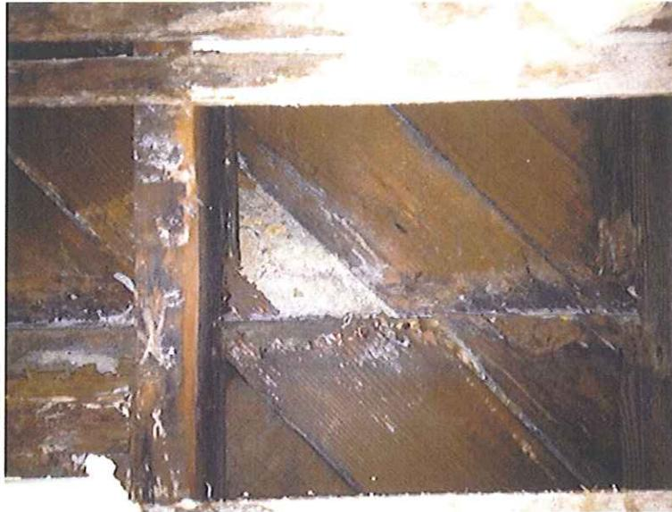
Photograph 5. South Wall Interior Showing Damaged Framing
