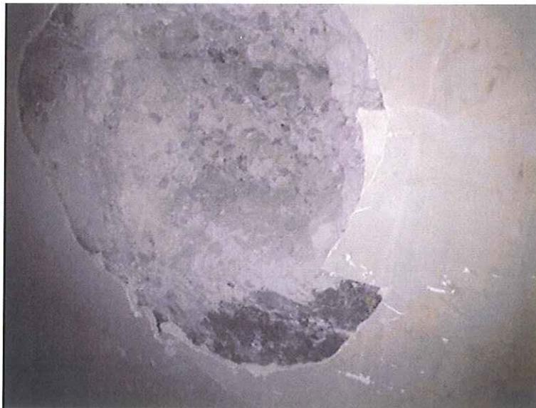
Photograph 12. Chipped East Wall in Basement Showing no Reinforcement in Concrete Wall
