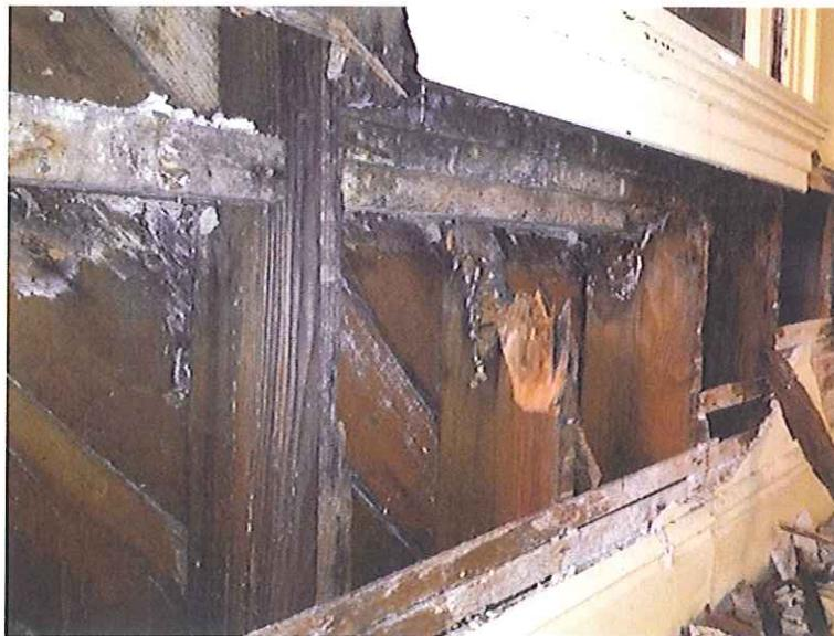
Photograph 4. South Wall Interior Showing Damaged Framing
