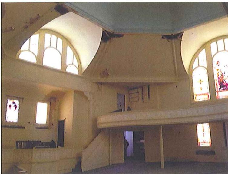
Photograph 10. Interior of Sanctuary Showing Water Damage
