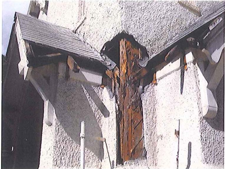
Photograph 1. Southeast Corner, Exposed Framing Below Stucco
