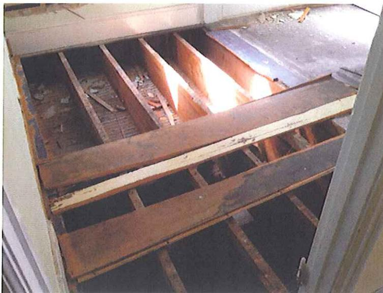
Photograph 14. Exposed Mezzanine Floor Framing
