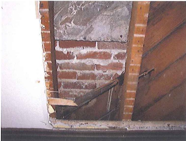
Photograph 8. South Wall Interior Showing Deteriorated Brick Masonry Veneer
