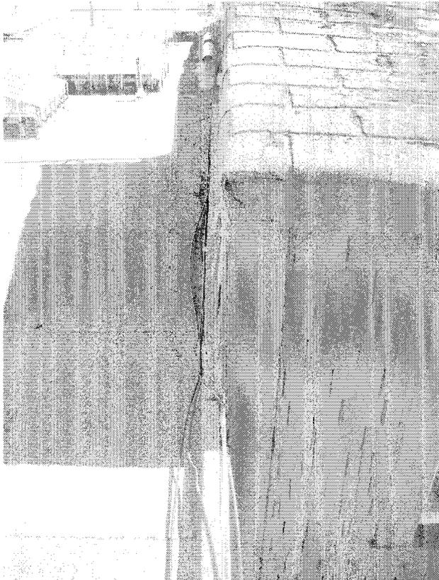
**Photo 11: This photo shows the rear addition leaning on the adjacent building to the north. Based on the survey by Geometrix, 1 McCormick is over the property line by almost 3".**
