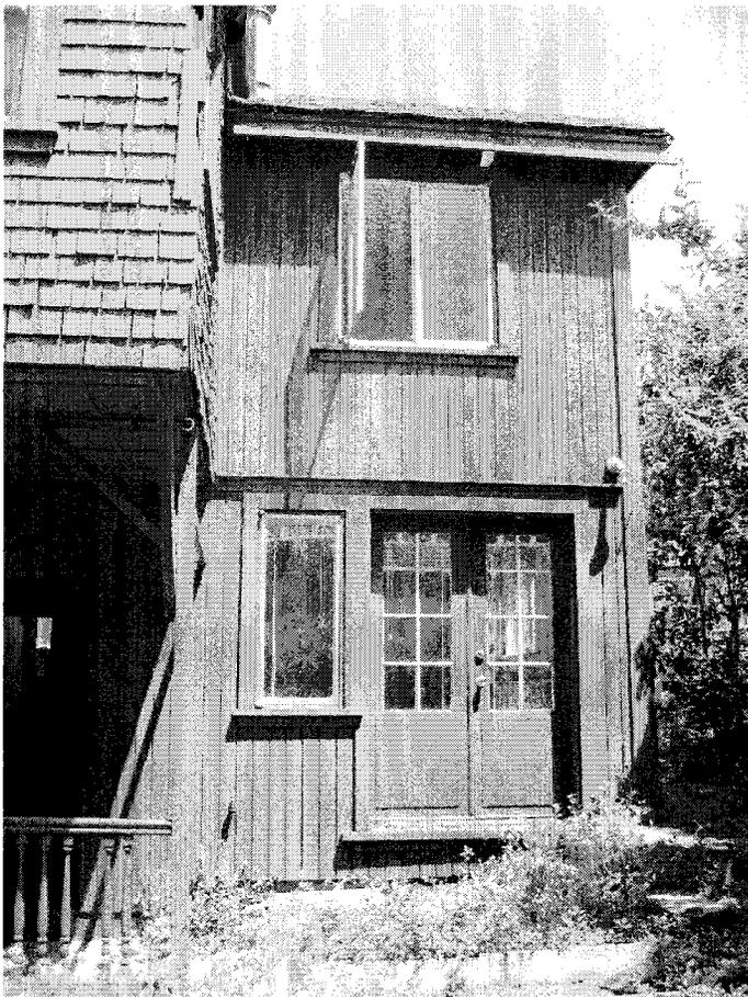
**Photo 26: Rear elevation illustrates different exterior sheathing materials.**
