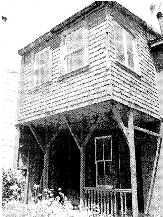
**Photo 7: The rear addition was added in 1947. Its primary support is the beam and three posts seen in the photo. This addition is also the location of the worst settlement in the building—as much as 6-inches lower than the zero point at the front door. This addition is also encroaching across the property line and leaning on the adjacent building.**
