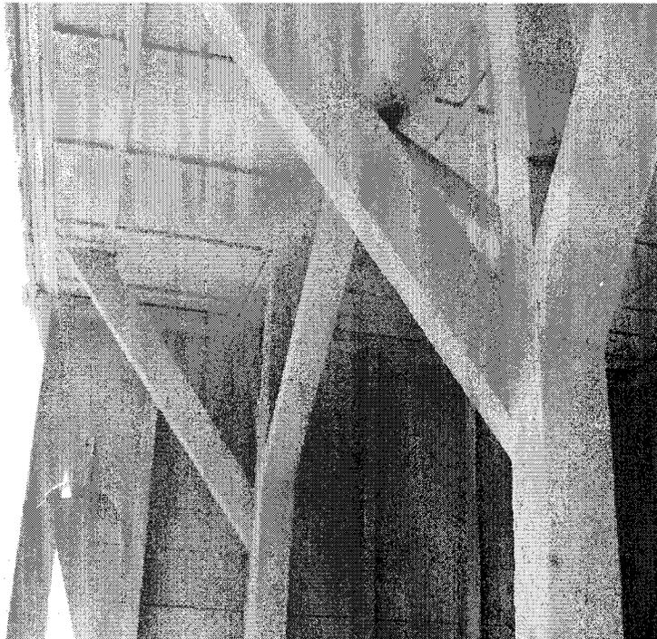
**Photo 8: Cantilever support beam connections are provided only by toe nails, i.e. nails that are driven at an angle to connect two members that are at an angle to each other.**
