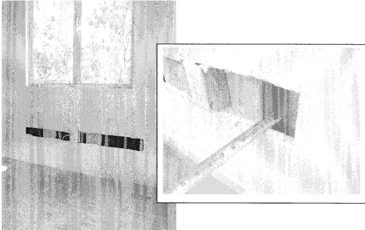
**Photo 9: Perimeter stud wall at second floor is framed with 1x2s.**
