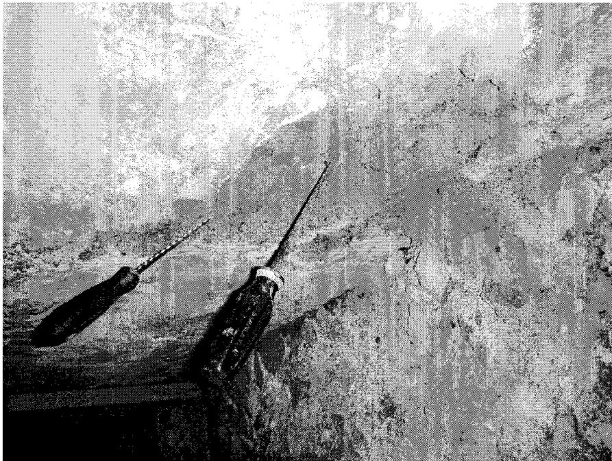
**Photo 24: Section of early rubble concrete foundation. The sizable chunks of brick in the aggregate will form large voids that may not be filled with sand and cement. The likely use of beach sand further shortened the life of the concrete to the point that one can now penetrate it with a screwdriver using relatively little force.**
