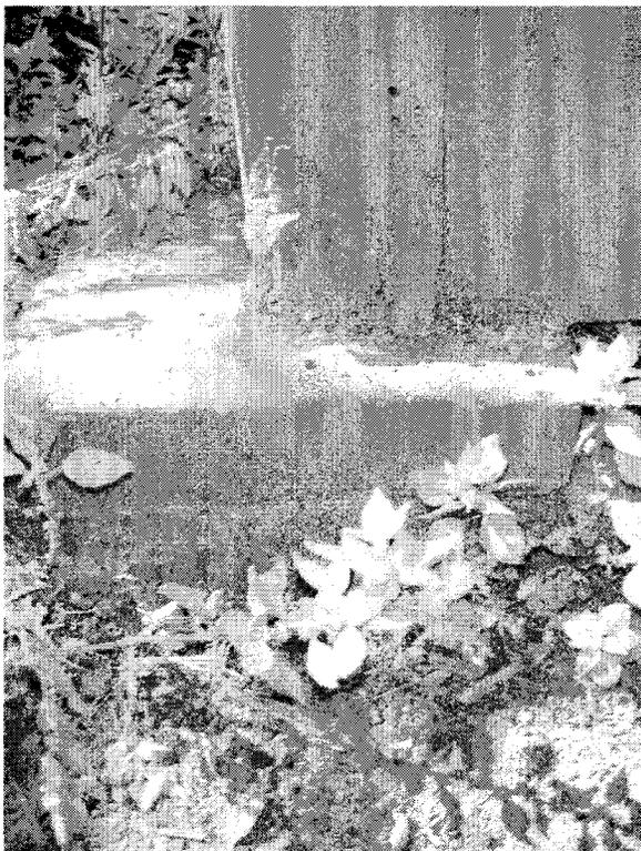
**Photo 20: This is an example of improper grade, showing how an inadequate separation between the earth and wood framing members can lead to rot at the foundation interface over time.**
