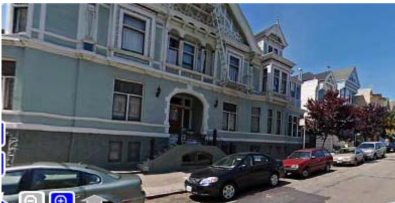
View north from intersection of Fell and Lyon Streets
