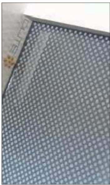
FRTTED GLASS PATTERN TO BE APPLIED TO THE NORTH FACADE SITE GLAZED OPENINGS ON THE THIRD AND FOURTH FLOORS. COLOR TO MATCH EXISTING BUILDING COLOR. PATTERN TO BE APPLIED TO THE EXTERIOR SIDE OF THE GLAZING FROM EXTERIOR AND ALLOW LIGHT AND SIGHT FROM INTERIOR.
