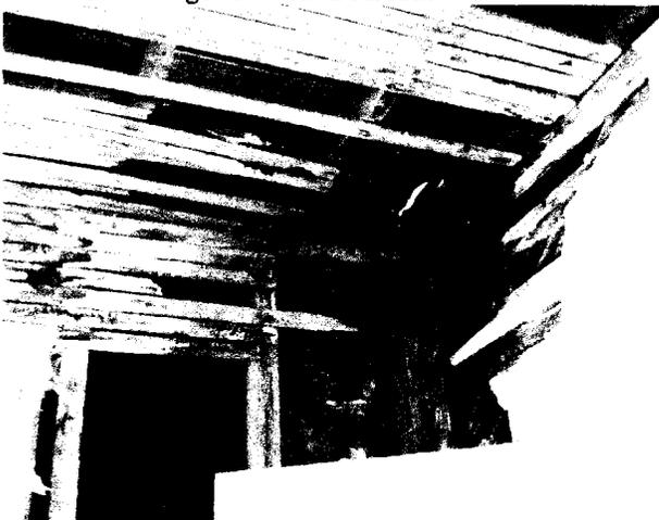
Photo 75: Severe Framing Deterioration at Sunroom
