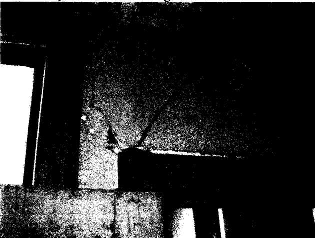
Photo 83: Shear & Settlement Cracks at Door
