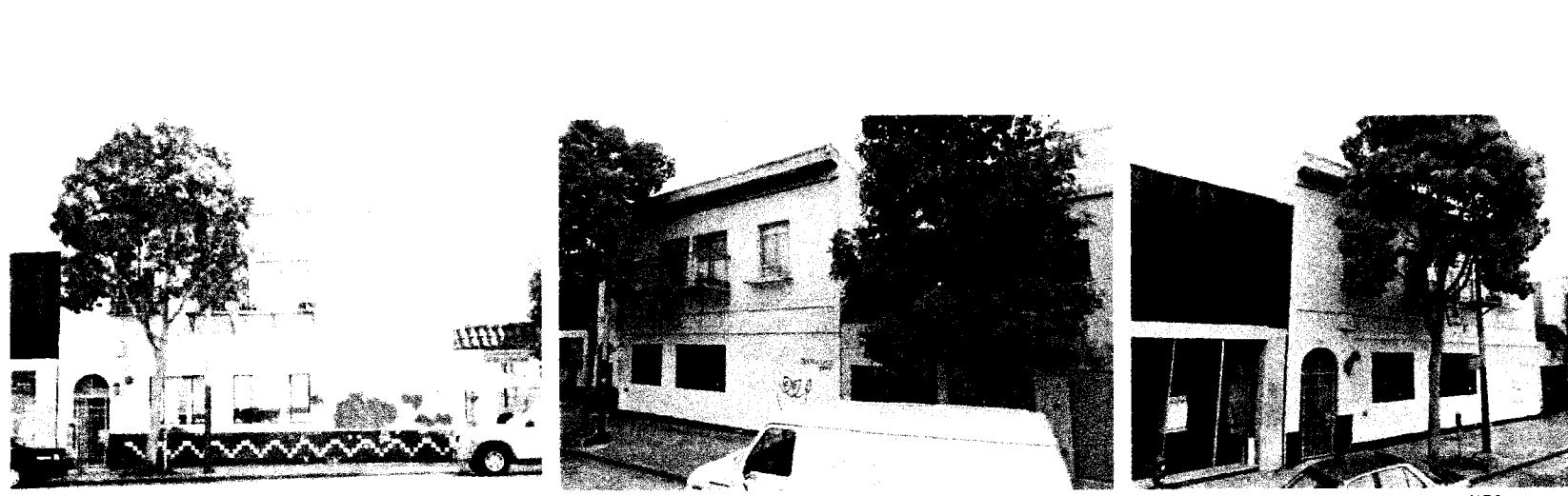
Existing Conditions Photos
