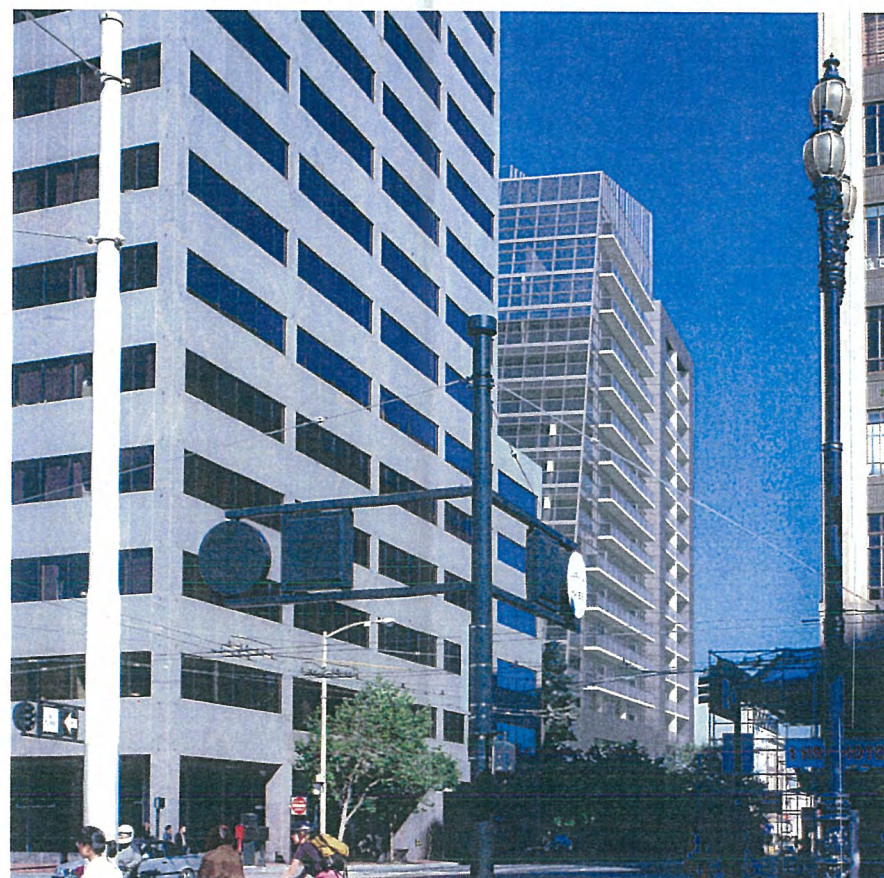
VIEW FROM MARKET STREET LOOKING SOUTH (E)
