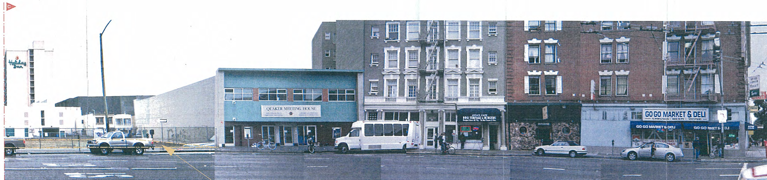
STREET-LEVEL ELEVATION OF NORTH-EAST SIDE OF NINTH STREET (C)
