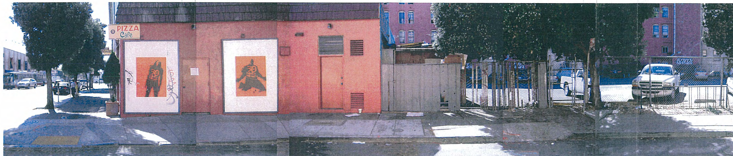
STREET-LEVEL ELEVATION OF SOUTH-WEST SIDE OF LASKIE STREET (B)
