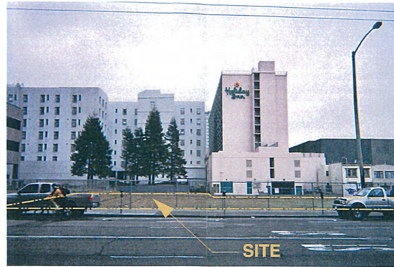
NORTH-EAST SIDE OF NINTH STREET (B)
