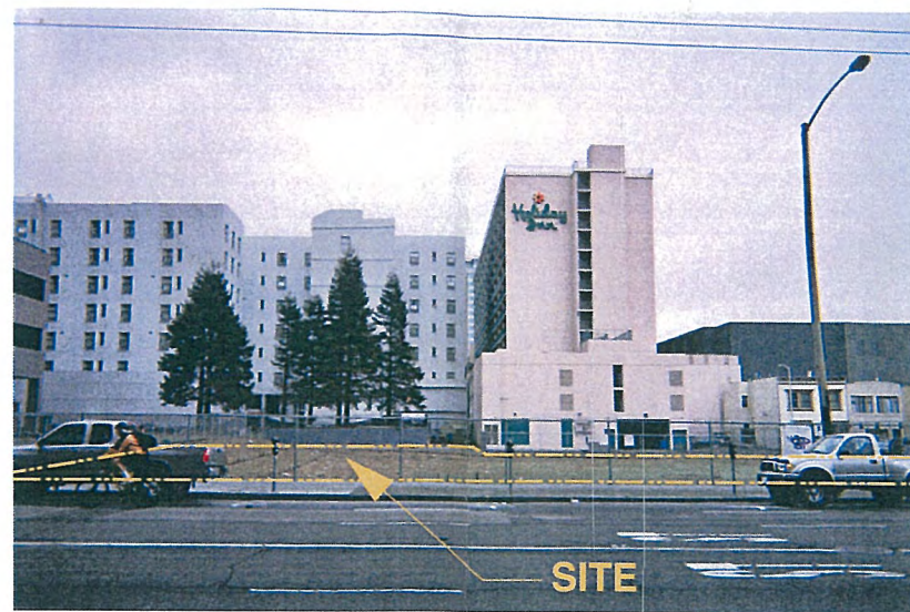
NORTH-EAST SIDE OF NINTH STREET (B)
