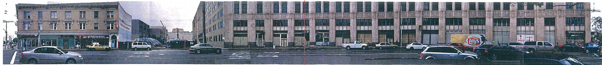
STREET-LEVEL ELEVATION OF SOUTH-WEST SIDE OF NINTH STREET (A) (COMBINED B+C BELOW)
