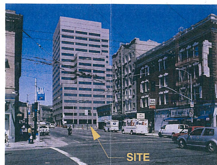
NORTH-EAST SIDE OF NINTH STREET - VIEW FROM MISSION STREET (C)
