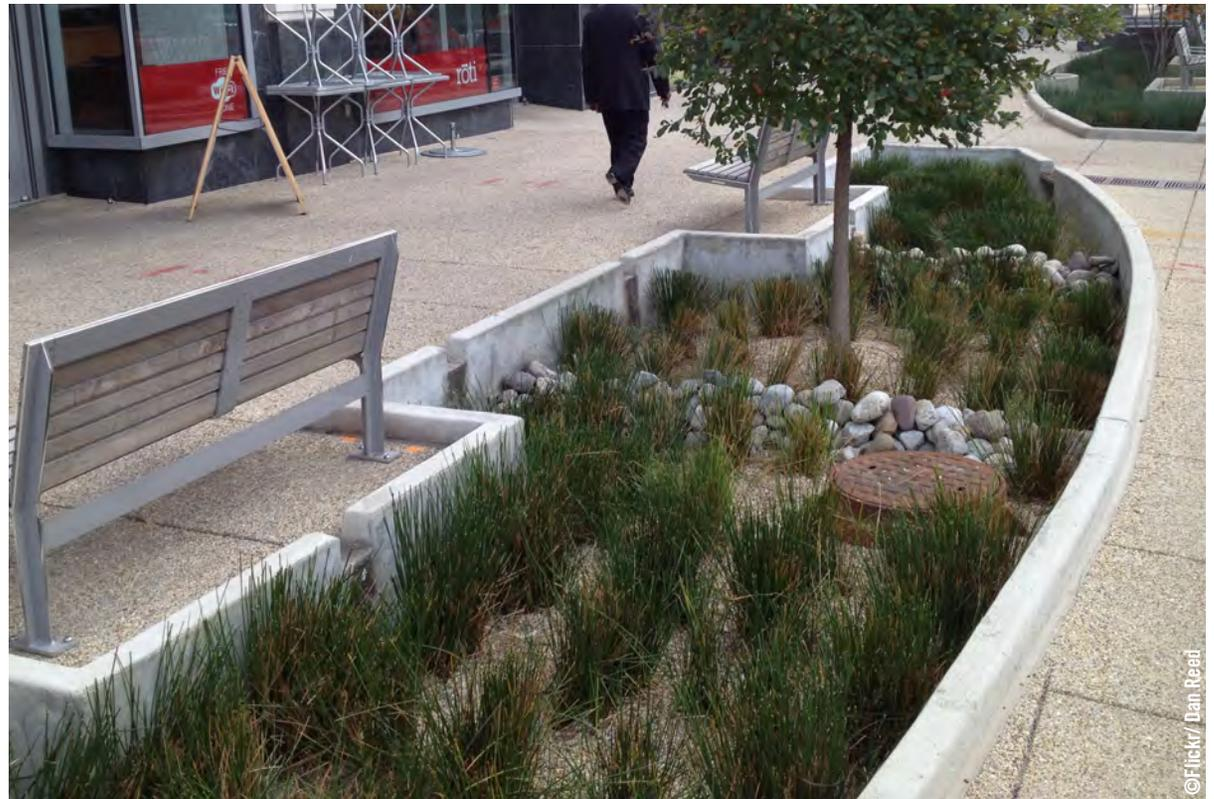
Fig. 9.4.2a Stormwater Planter
