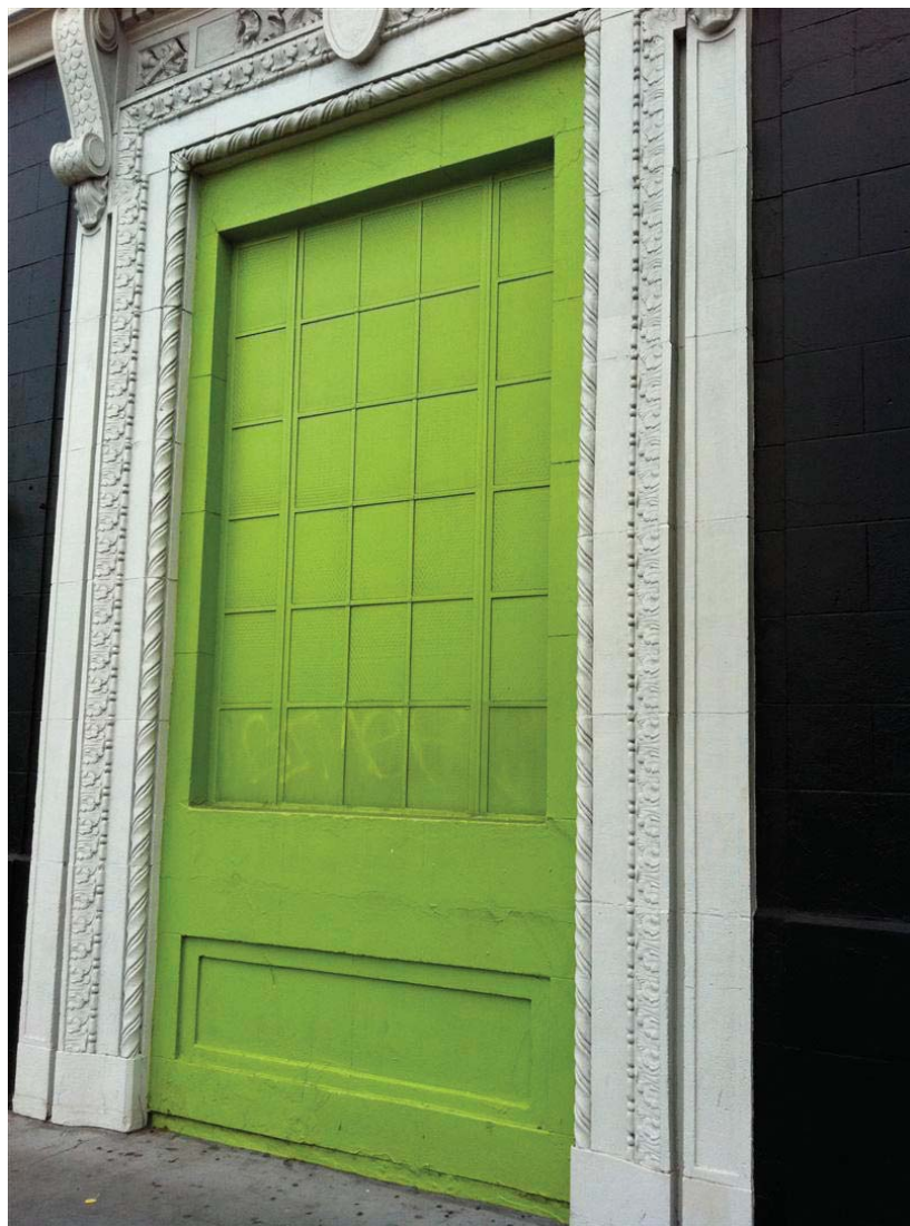
BRANNAN STREET WESTERN PORTAL
