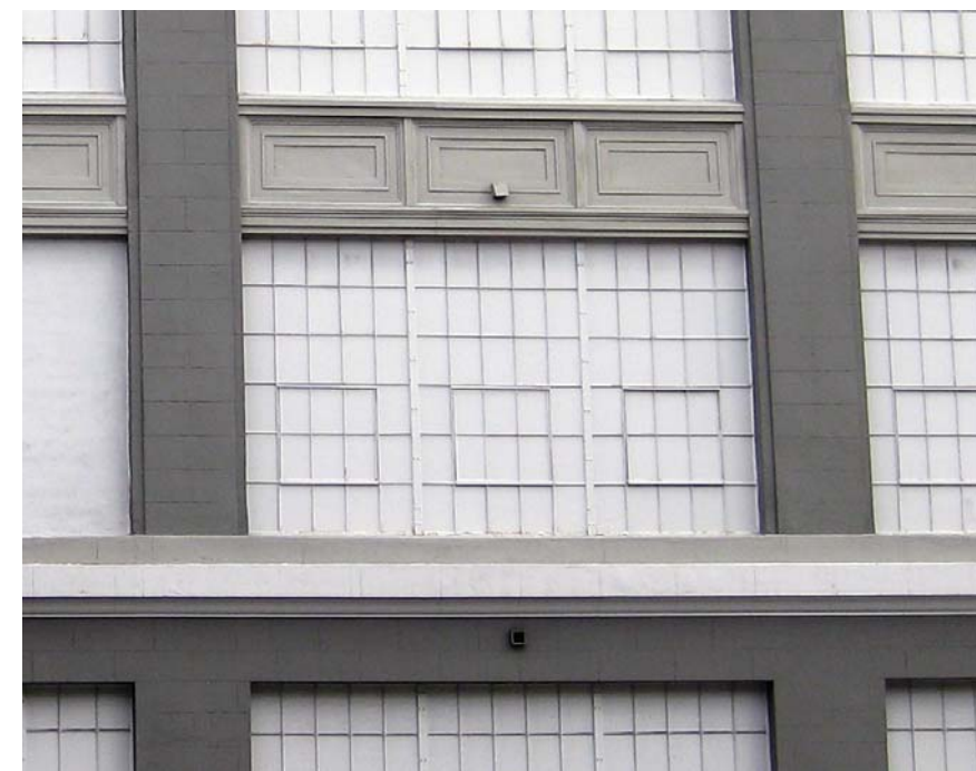
TYPICAL EXISTING WINDOW
