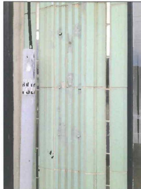
PHOTO A: DAMAGED TILE DETAIL AT LEFT PILASTER
