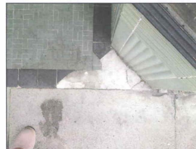
PHOTO C: DAMAGED TILE DETAIL AT HISTORICAL ENTRY
