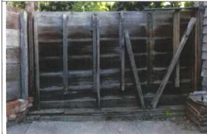
North exterior wall. Note the level floor line at the bottom of the original framing studs.
