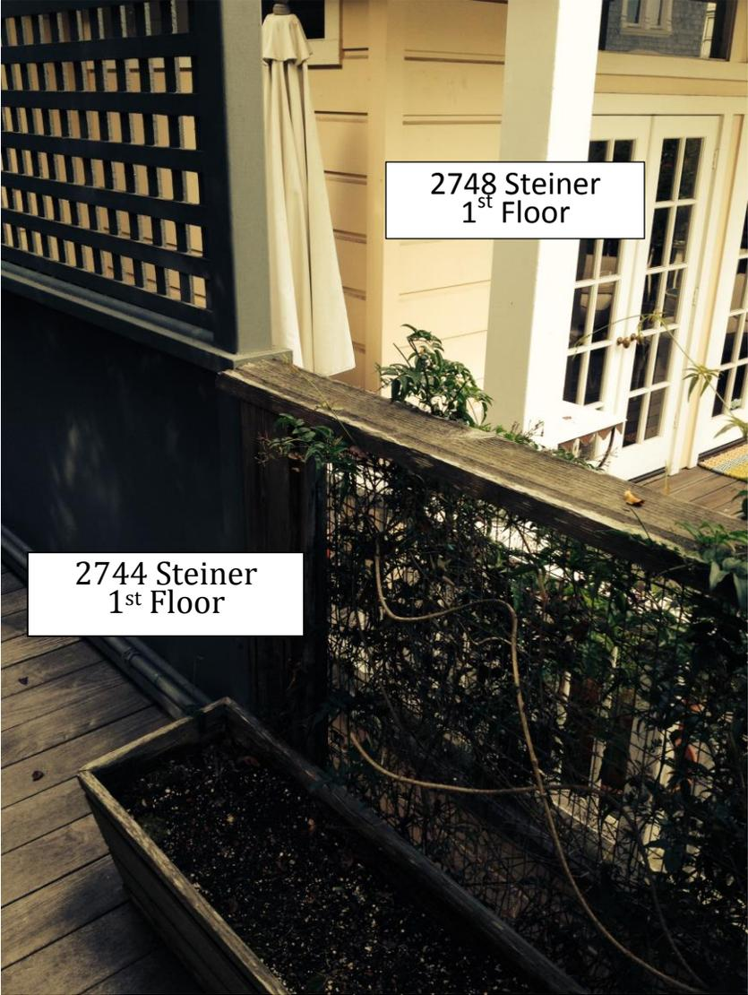
THE GRADE DIFFERENCE BETWEEN 2744 STEINER, 1<sup>ST</sup> FLOOR AND 2748 STEINER, 1<sup>ST</sup> FLOOR IS ONLY 2'-1"
