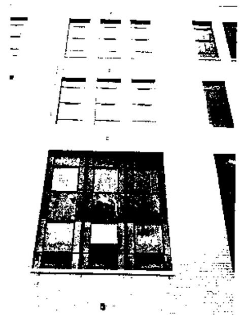
Figure 4. Among the retained and repaired original windows were these large units on the second floor level. Photo: Bruner/Cutt & Assoc., Inc.
