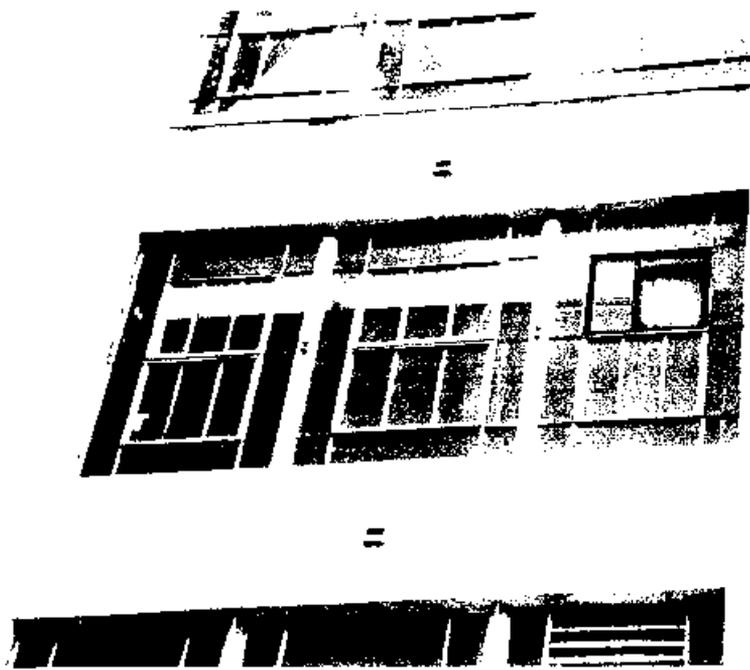
**Figure 1.** Many of the original Lupton windows incorporated a pair of stacked ventilators that projected outward. The vents were centrally located within a multi-light frame each of which was set either individually or in groups of two or three. Photo: Bruner/Cott & Assoc., Inc.
