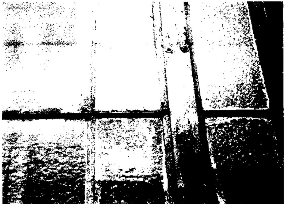
**Figure 2.** Narrow sightlines, ventilator weathering flanges and mullion boltheads were all distinguishing features of the original steel windows. Photo: Bruner/Cott & Assoc., Inc.
