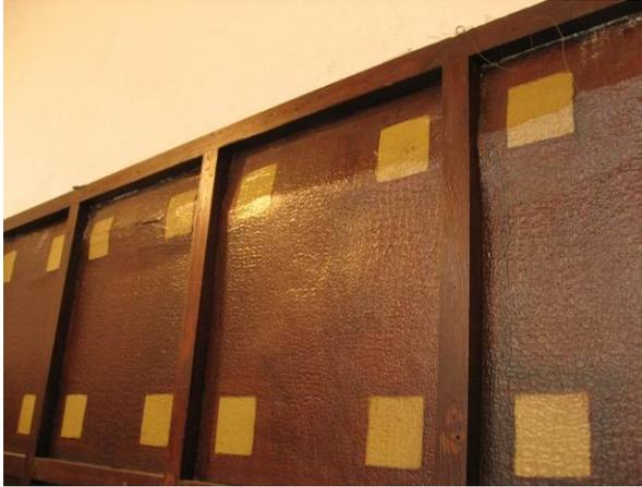
*Detail of leather paper wall cladding. Note damage.*
