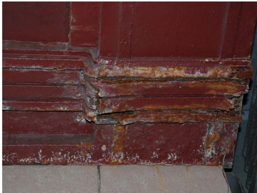
42. Detail of existing canopy on Market Street, showing deterioration of the underside
