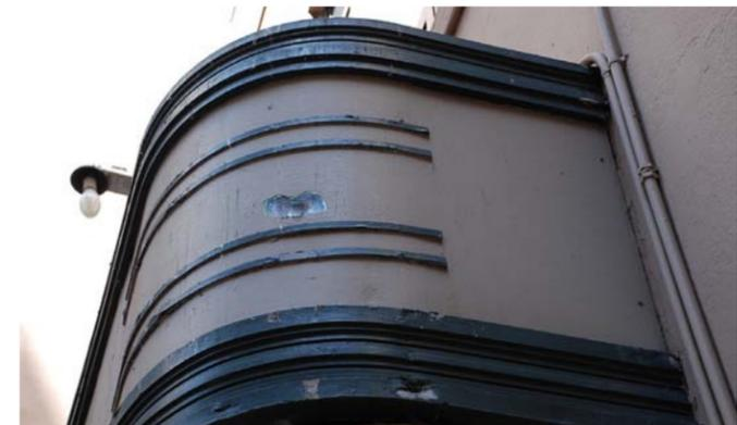
44. Detail of existing canopy on Stevenson Street, showing deterioration of the sheet metal face
