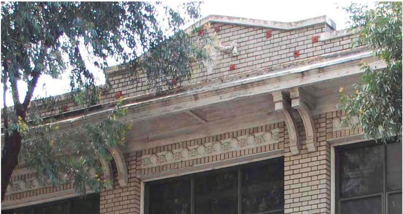
Detail of parapet, cornice, brackets, and frieze ornament. The windows have replacement metal sash set within original wooden frames.
