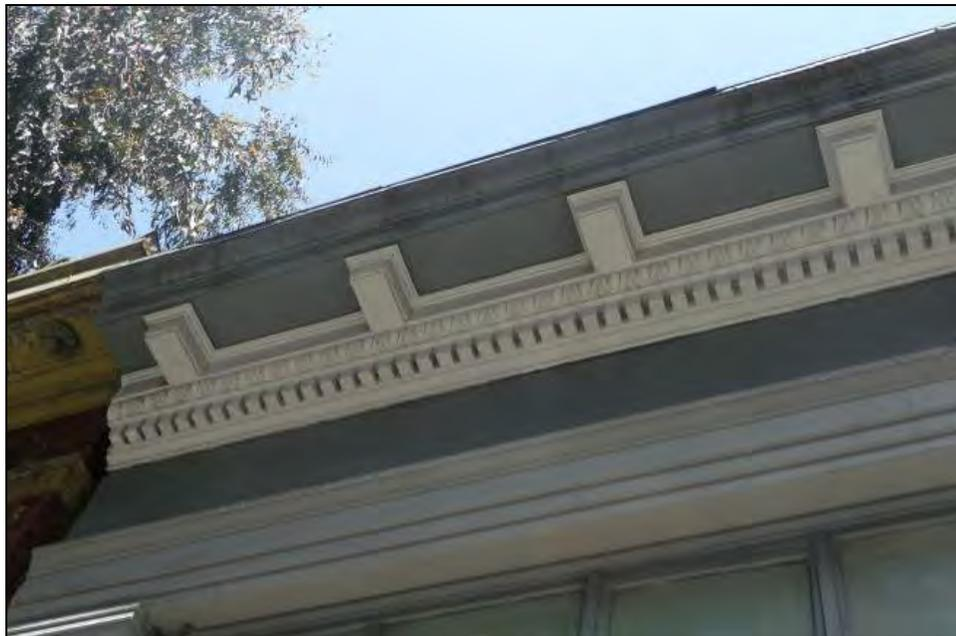
**Photograph 4:** 1634-44 Pine Street. Detail of profiled cornices, courses of egg-and-dart, dentils, blank frieze.
