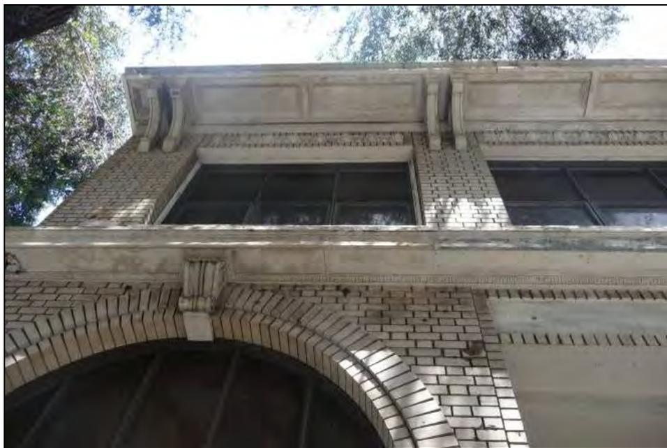
**Photograph 12:** 1670 Pine Street. Detail of parapet and cornices.
