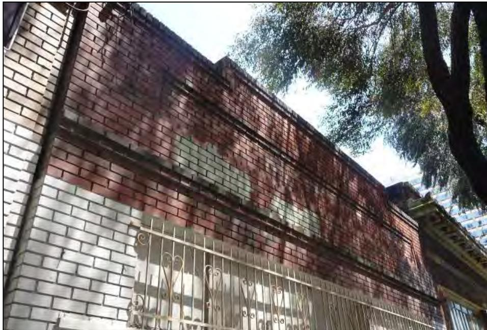
**Photograph 8:** 1656 Pine Street. Detail of brick façade, parapet, panel, and cornice.
