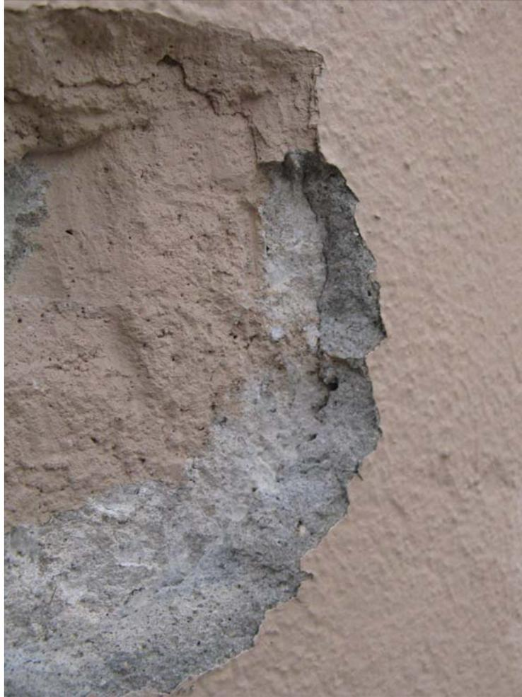
**Sample 3 detail: separation of old bedding mortar and added cement stucco**
