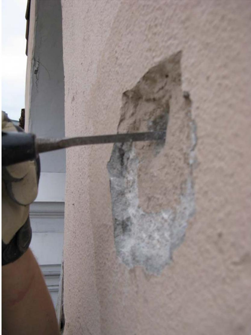
**Sample 3: Cutting into concrete substrate**
