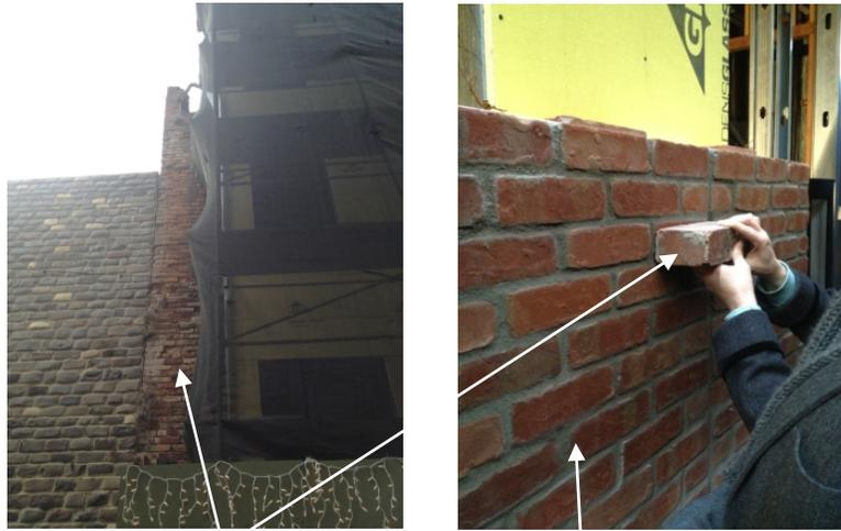
Original brick and mock-up of brick veneer.
