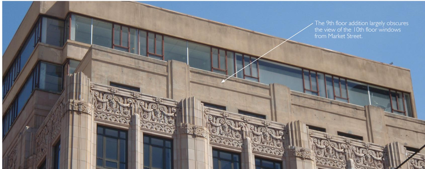
The non-historic ribbon windows at the 10th and 11th floor will be removed and replaced. The existing windows exhibit rust and are generally in poor condition and have poor thermal qualities. The 11th floor windows will be replaced with new windows that are the same height and have a similar configuration. At the 10th floor, the window sill will be lowered from 4'-6" to about 3'-0" to improve the view for this tenant space.
