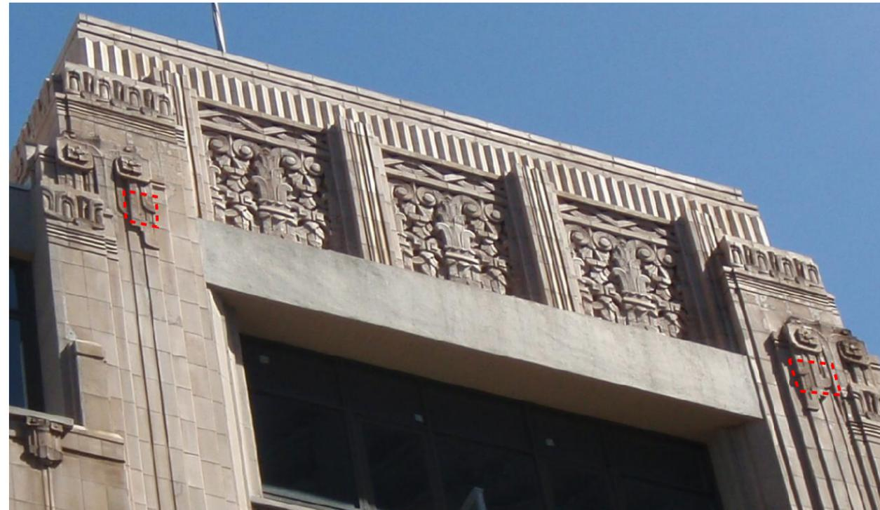
Terra cotta (shown in dashed rectangle) is to be removed and salvaged to allow for the installation of window washing equipment
