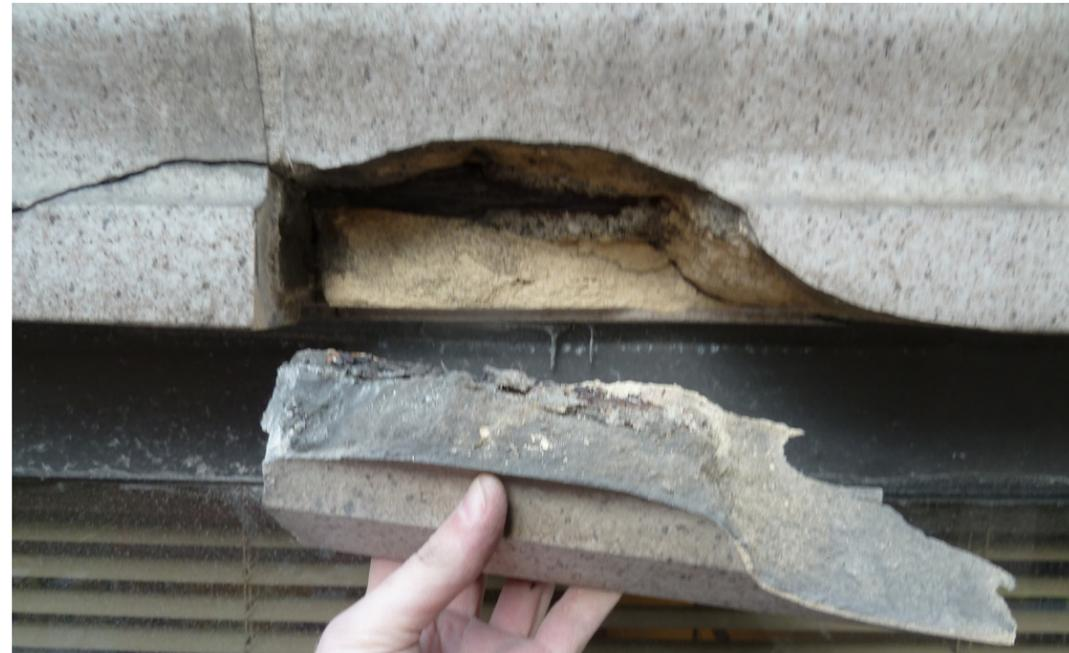
Severe spalling of terra cotta unit and corrosion of anchors
