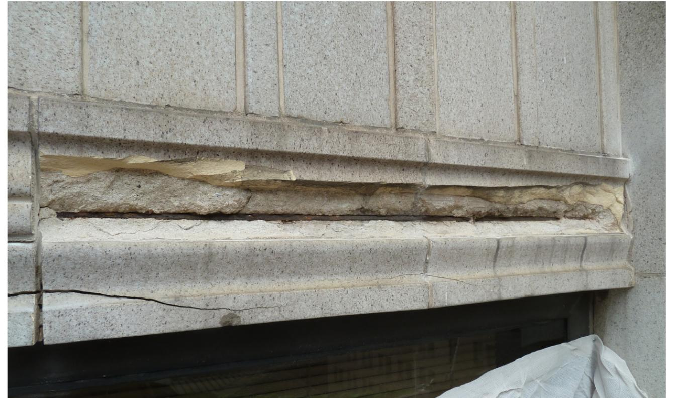
Severe spalling of terra cotta unit and corrosion of steel angle
