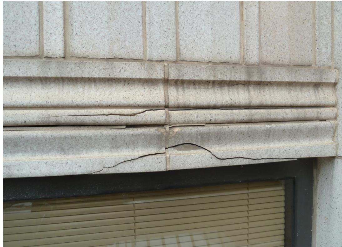
Severe cracking at window header terra cotta unit
