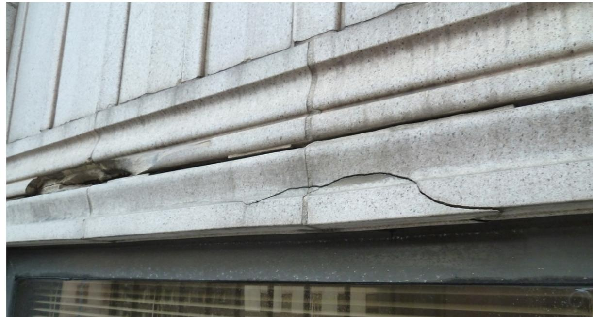
Severe spalling of terra cotta unit and horizontal cracking
