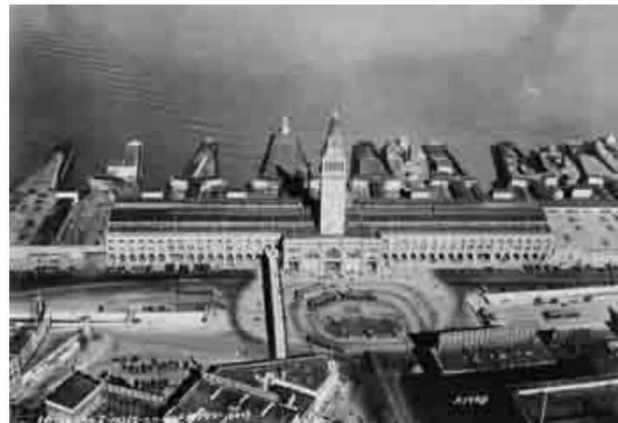
View of historic intermodal terminal, showing the vehicular subway, the transit turn-around and the elevated pedestrian bridge and multiple ferry slips, 1930s
