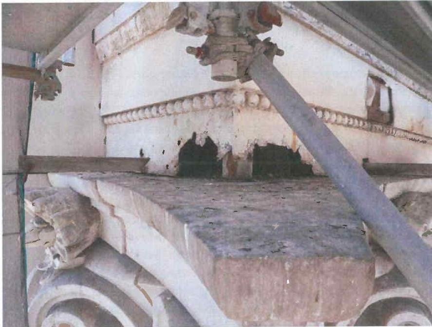
Detail of deterioration and holes where birds enter as well as steel outriggers atop column capitals
