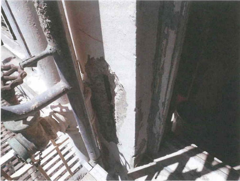
Typical spalling at parged concrete
