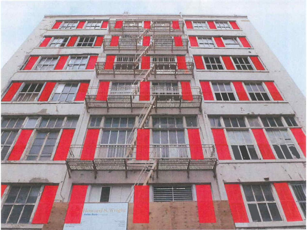
View of Stevenson Street façade looking up showing typical locations of double hung sash being replaced with new wood double hung sash. (Replaced sash areas shown in **RED**).
