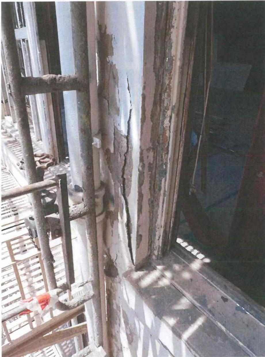
Typical spalling at parged concrete
