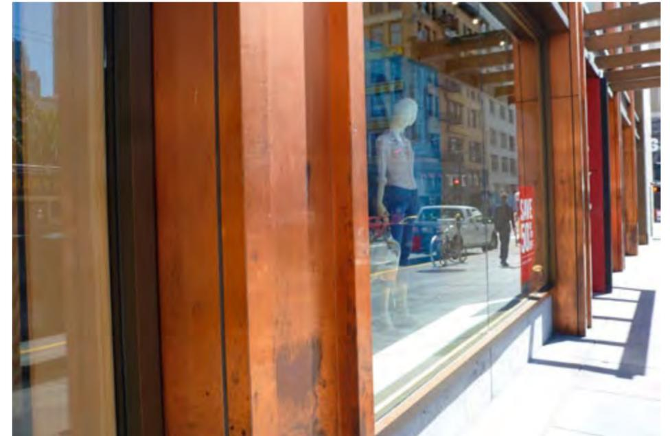
**D. Detail of the copper I-beams on the primary facade of the Levi's store.**
