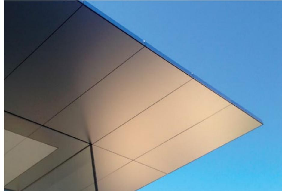
**Bead Blasted Stainless Steel Roof Overhang**
