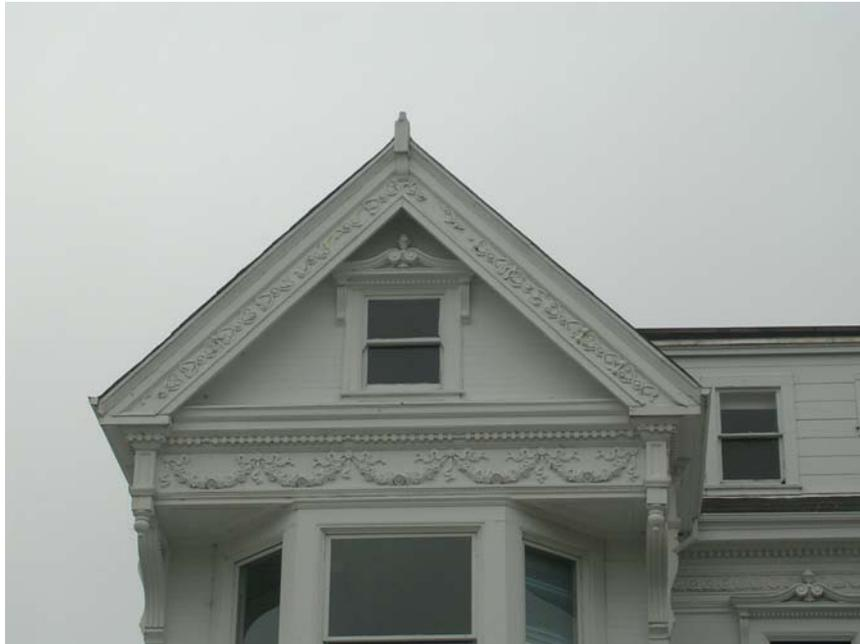
Image 22. The attic window with swan-neck pediment sits within the Queen Anne Style gable supported by an Ionic entablature with decorative festoons at the frieze. Knapp Architects, digital photograph, 2009.
