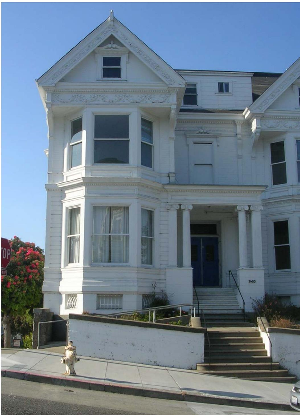
Image 21. Character-defining projecting bay with decorative gable over two-story bay window and basement window at coursed concrete base. Knapp Architects, digital photograph, 2009.
