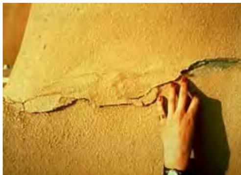
A waterproof coating is an inappropriate substitute material to apply to adobe as it seals in moisture and may result in spalling. Photo: NPS files.
