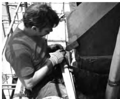
patches, cool and damp conditions). At temperatures below 50F (10 C), use of *RL-6* winter grade latex is recommended to accelerate curing.
