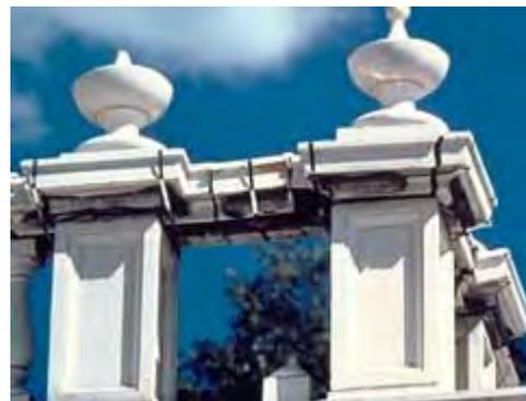
Exposed or freestanding terra-cotta detailing (parapets, urns, balusters, etc.) have traditionally been subjected to the most severe vicissitudes of deterioration as a result of freezing temperatures and water. Photo: NPS files.
