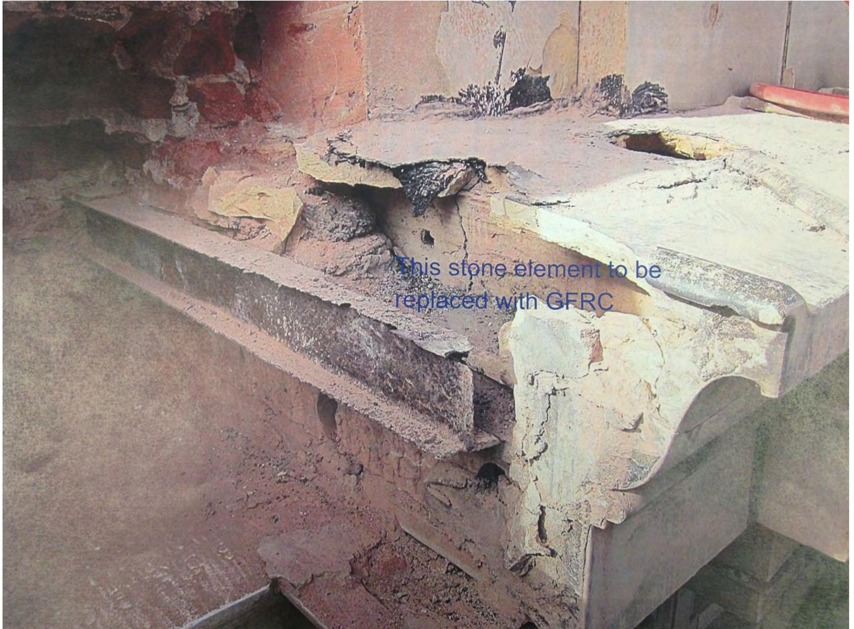
This stone element to be replaced with GFRC
