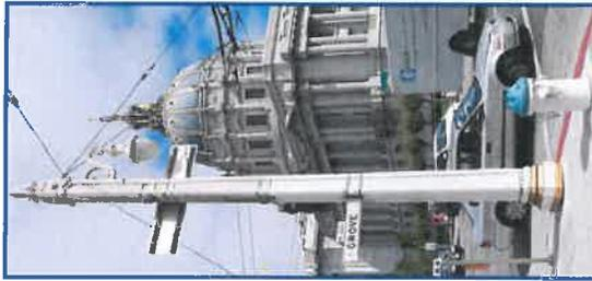
Van Ness trolley pole with single pendant and high pressure auxiliary water supply hydrant
