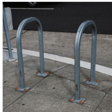
Bike rack - metal staple style, installed incorrectly along Grove St
