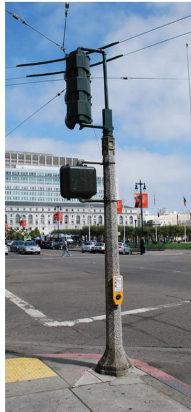
Modified aggregate concrete post with traffic signal
