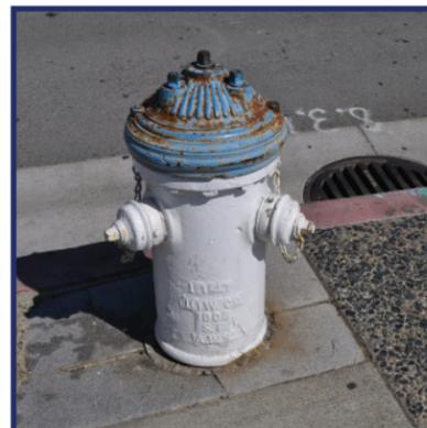
High pressure auxiliary water supply hydrant at Larkin St
