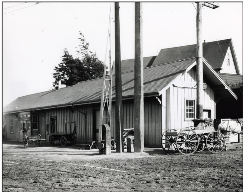
The Southern Pacific’s Ocean View station was a passenger stop as well as a major siding with a spur accommodating 91 railroad cars. The station was a one story, gable roof, wood building typical of the Southern Pacific’s smaller train stations of the period and is no longer extant. Nothing remains today that suggests Ocean View’s railroad past. (Walter Rice and Emiliano Echeverria, *When Steam Ran on the Streets of San Francisco* (Forty Fort, PA: Harold E. Cox, 2002), 69
