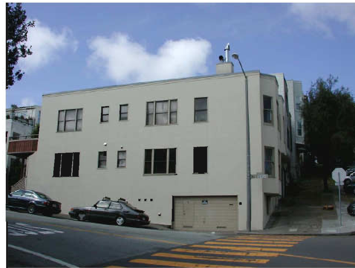
4 VIEW OF BUILDING AT SOUTHWEST CORNER N.T.S.
