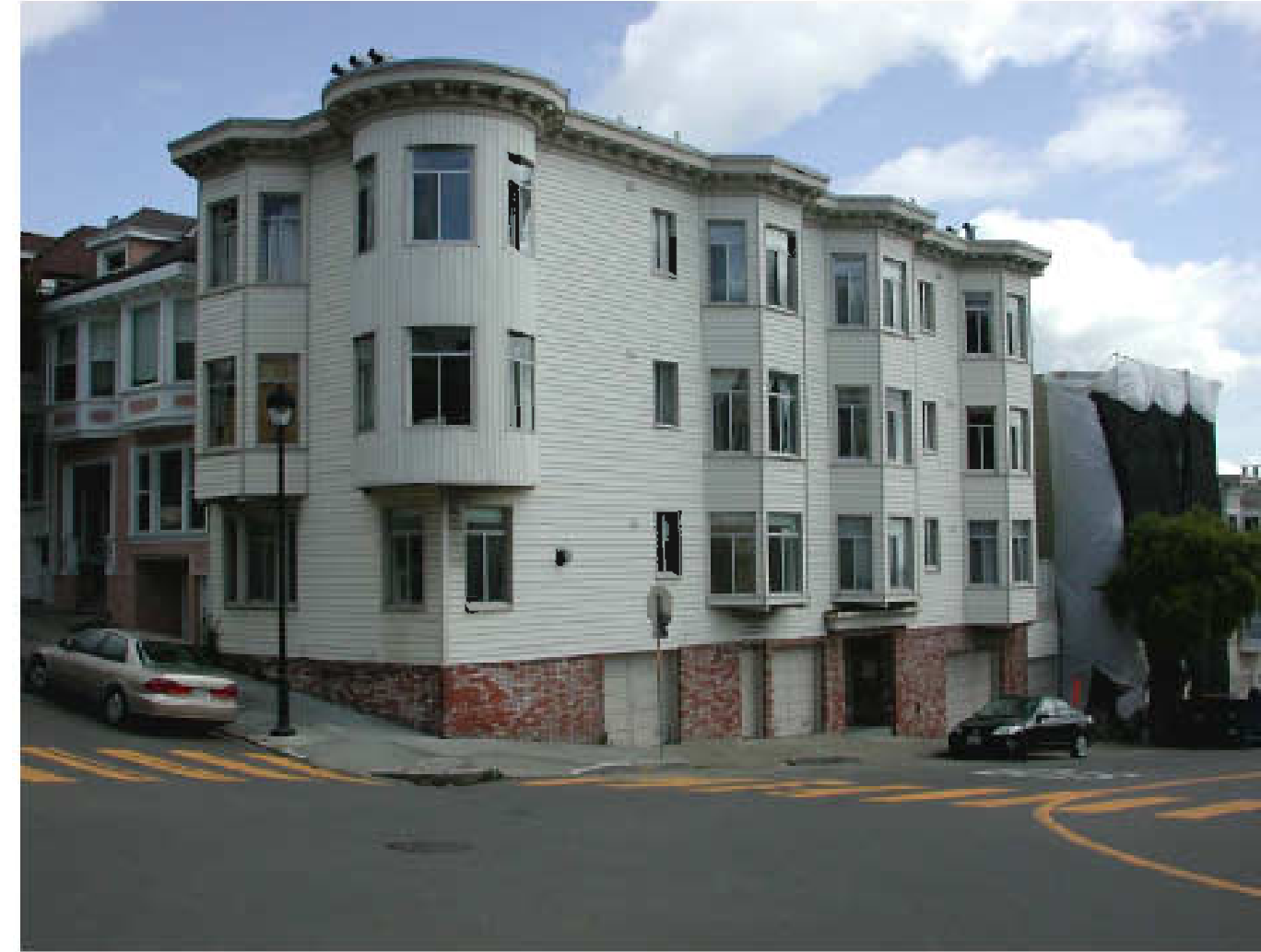
5 VIEW OF BUILDING AT NORTH EAST CORNER N.T.S.
