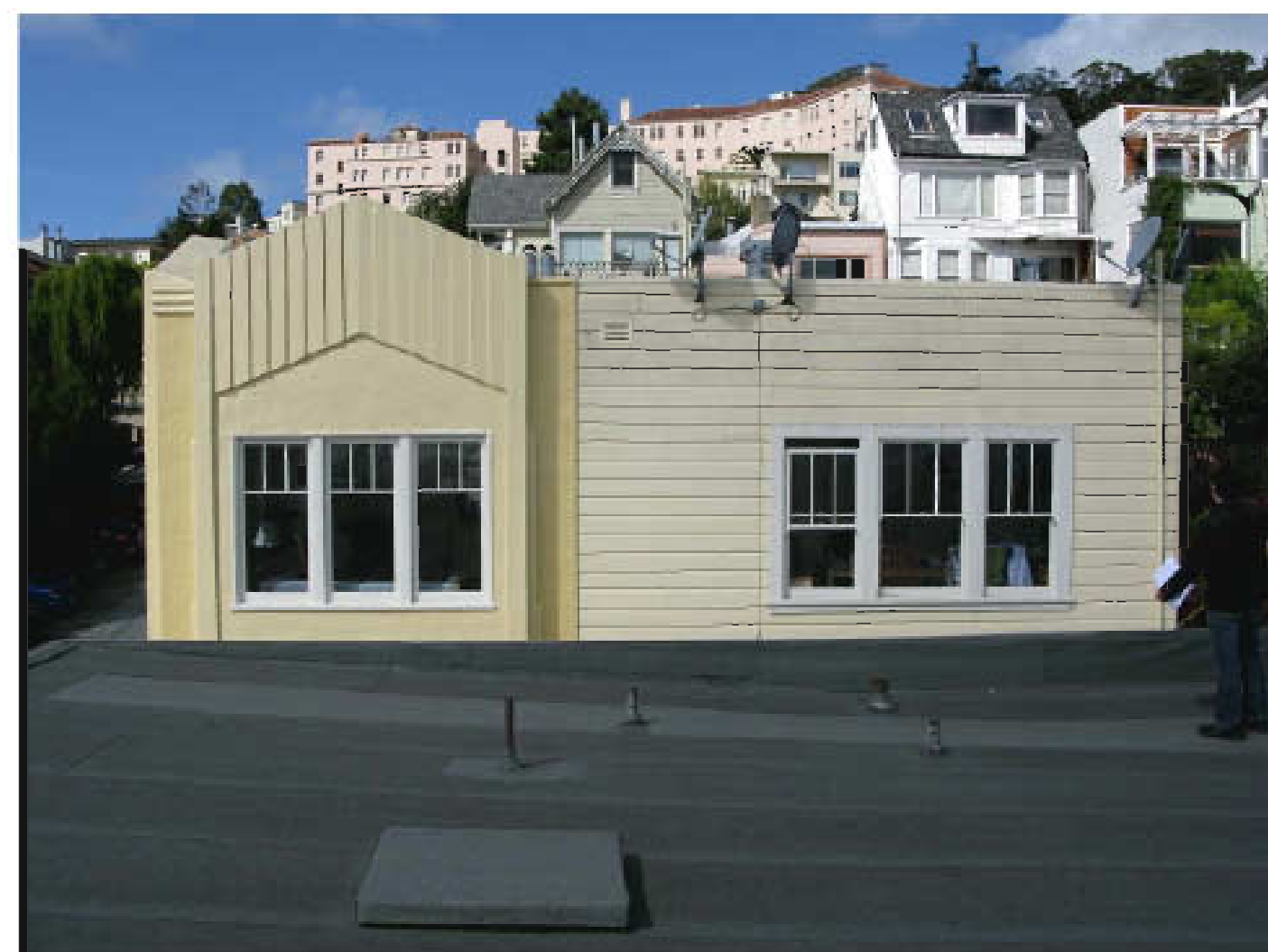
7 WEST VIEW OF ADJACENT PROPERTY FROM ROOF N.T.S.
