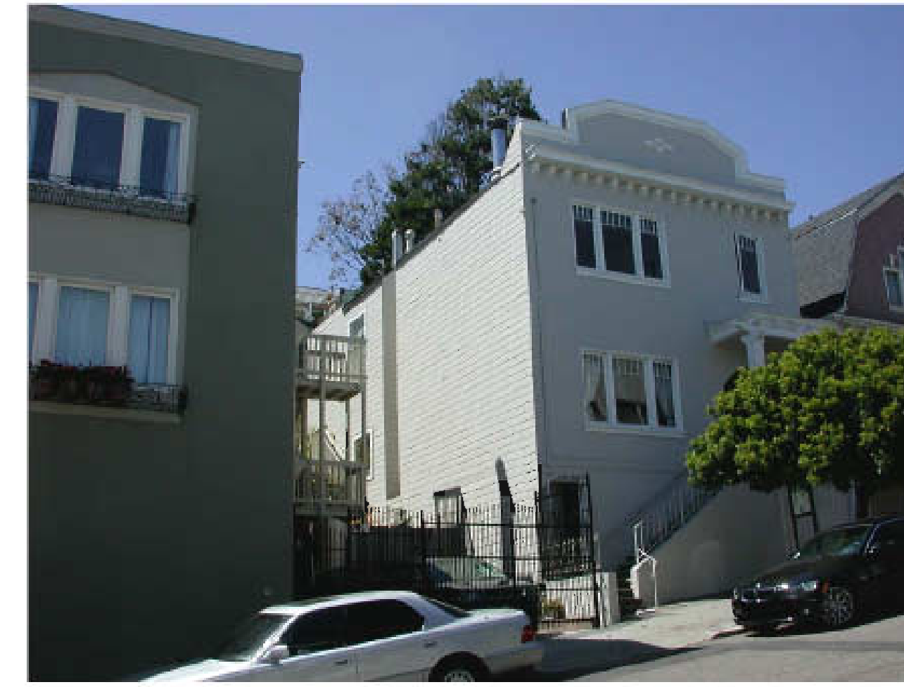
3 VIEW OF ADJACENT BUILDING ON ALPINE N.T.S.
