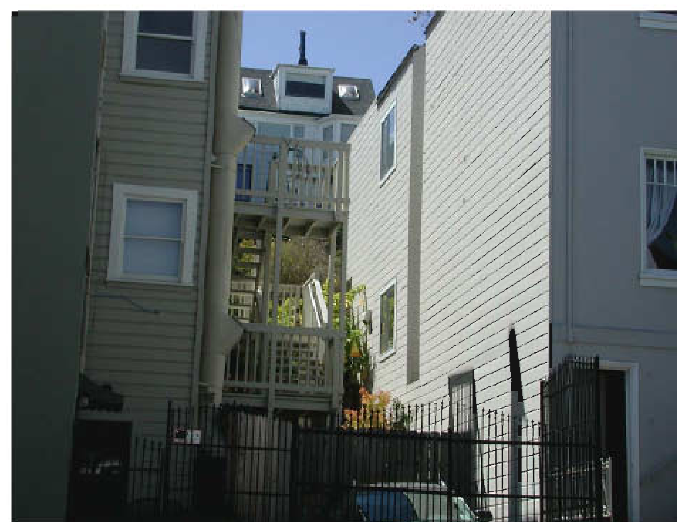
8 NORTH VIEW OF ADJACENT PROPERTY N.T.S.
