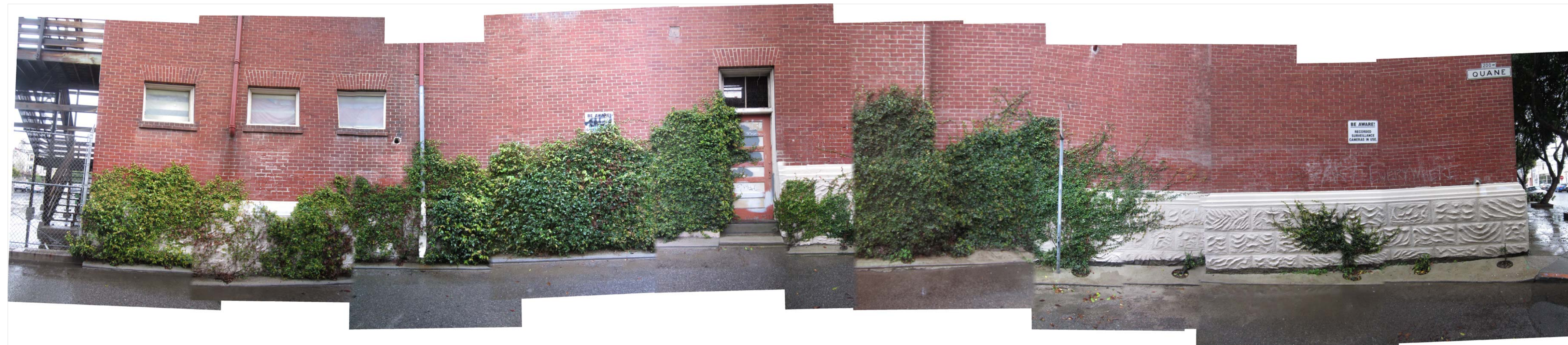
EAST SIDE OF QUANE ALLEY ACROSS FROM COTTAGE SITE
